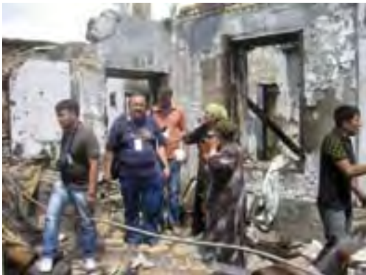
Burned out buildings in Osh.
