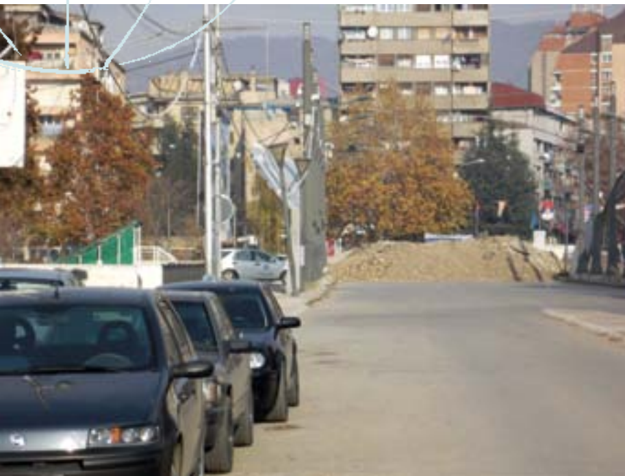
Blocked bridge in Mitrovica
